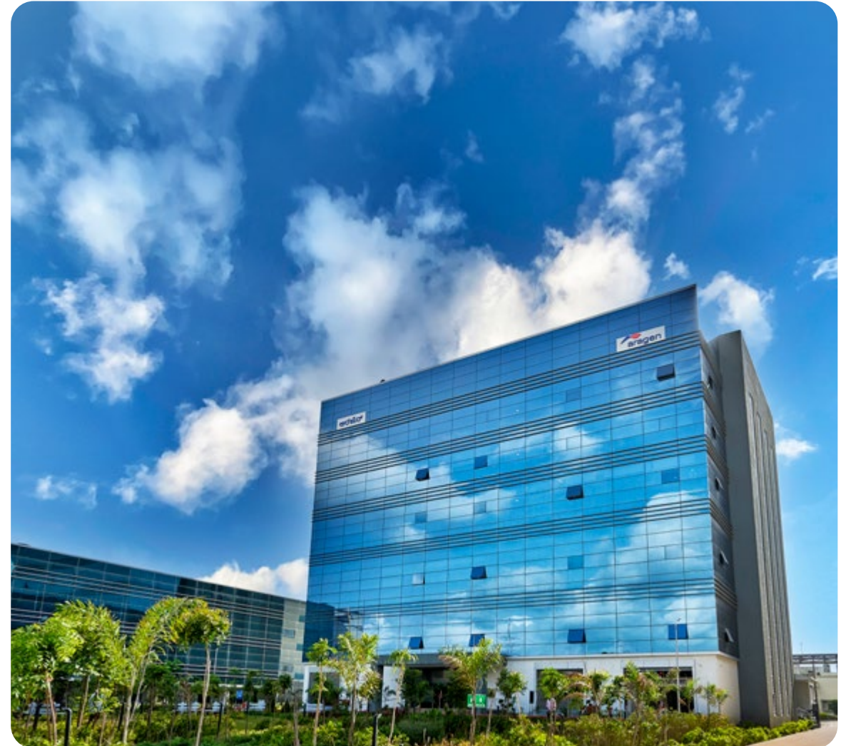
Impressive sustainable infrastructure of Biologics manufacturing at Bengaluru
