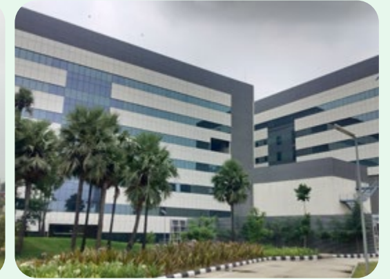
MLR-4 & MLR-5 buildings at Mallapur facility
