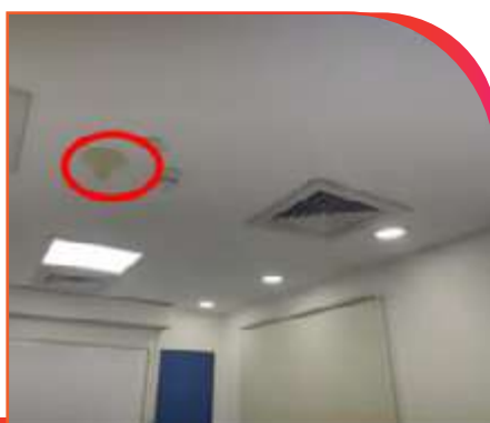
Installation of Motion Sensors
