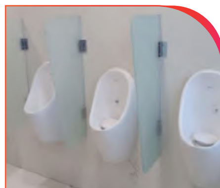
Installation of Waterless Urinals
